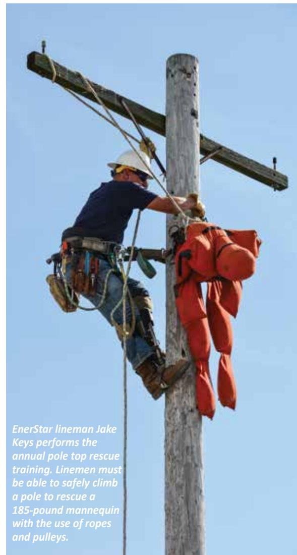
*EnerStar lineman Jake Keys performs the annual pole top rescue training. Linemen must be able to safely climb a pole to rescue a 185-pound mannequin with the use of ropes and pulleys.*
