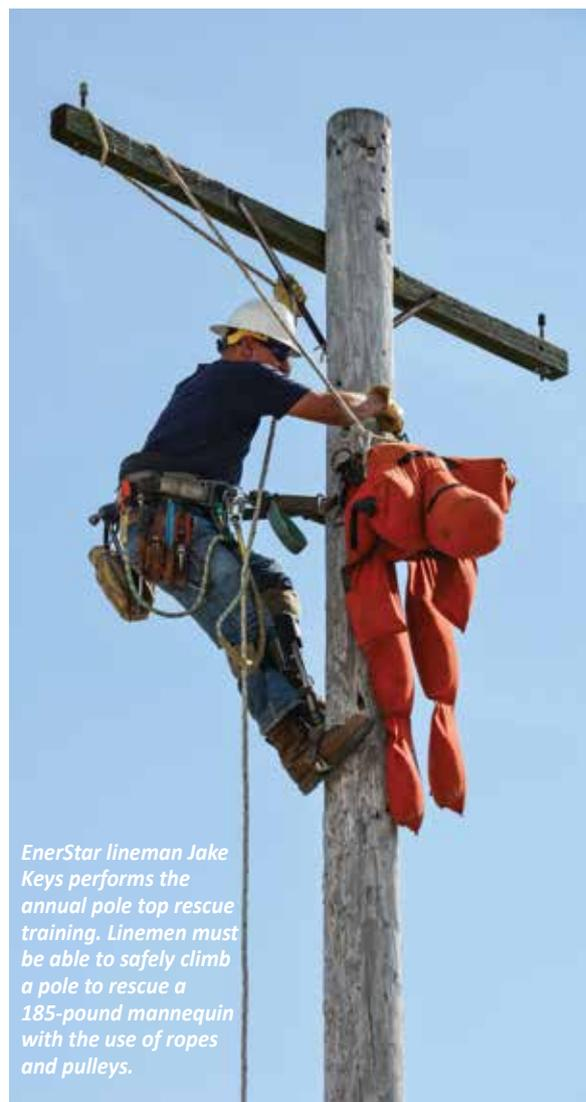
*EnerStar lineman Jake Keys performs the annual pole top rescue training. Linemen must be able to safely climb a pole to rescue a 185-pound mannequin with the use of ropes and pulleys.*
